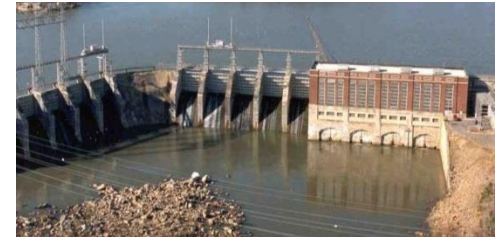
Wylie Hydro Station
